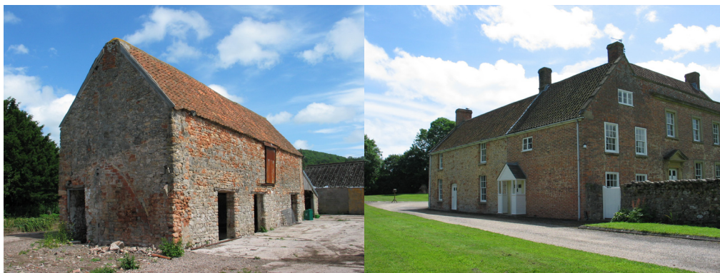
Dulcote West Mill, drying house, 2005
