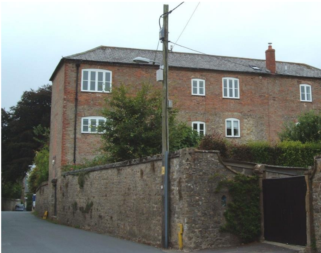
Whitcombe Flax Factory showing bottom two stories stone and extension top storey in brick.
