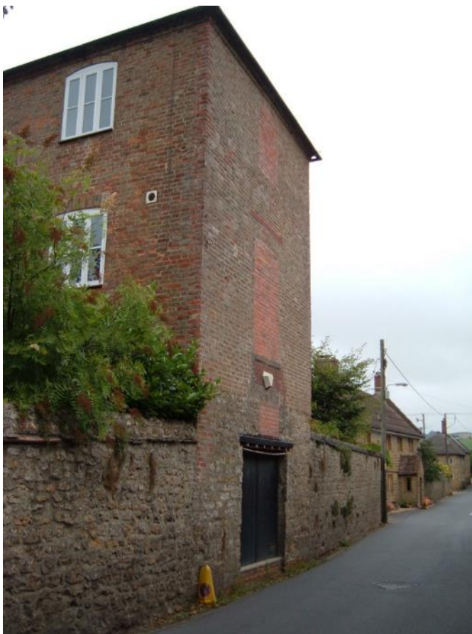
Road end of Whitcombe Road Factory. The bottom door was probably for cart storage. The upper two doors for loading carts from the factory. The road width here is 12 ft, wide enough for a cart to turn round?
