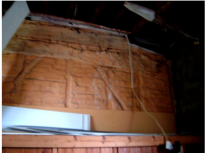
Original beams and in-fill brickwork
