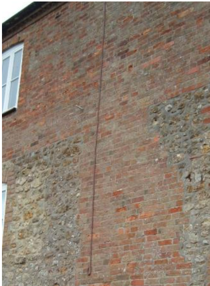
Flue through stonework.
