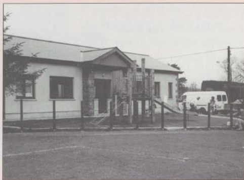
Tavernspite village hall: If WCVA's bid to the Millennium Commission gets the go-ahead, many halls in rural communities could benefit from similar renovations.
